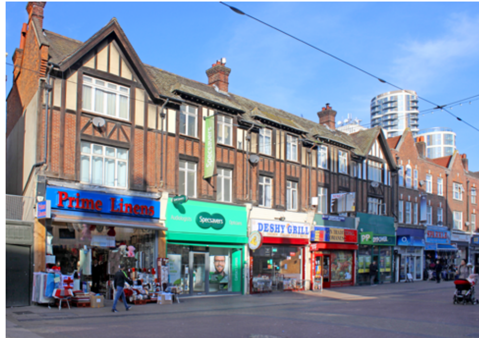
Typical three-storey terraced buildings along East Street.
