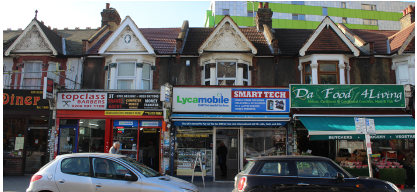
Nos. 40-46 Ripple Road are positive buildings, despite later insensitive modern shop fronts and signage
