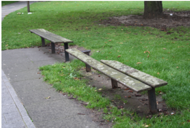
Dilapidated seating in Abbey Green.
