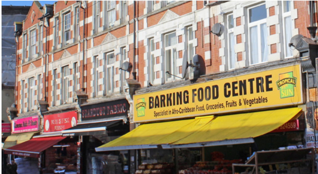
Satellite dishes attached to principal elevations of buildings in the conservation area.
