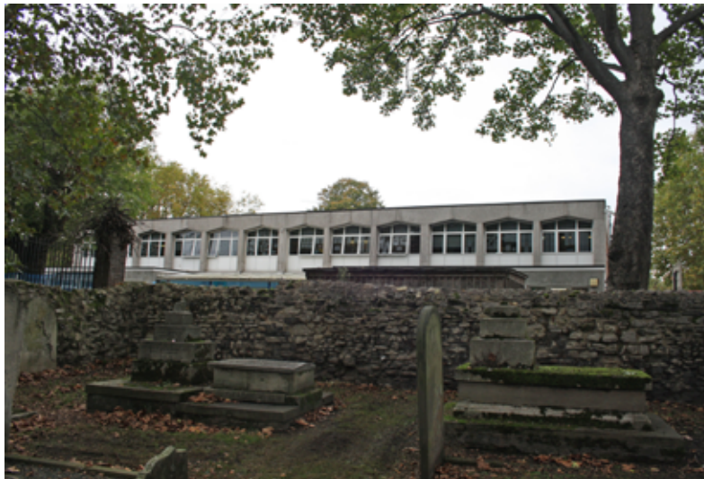
St Margaret's Primary School is a neutral building.
