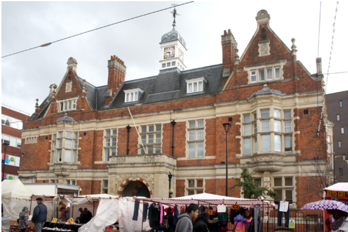
Barking Magistrates' Court in East Street was originally the Local Board Office and a Free Library.
