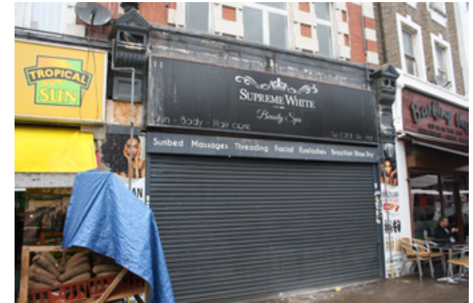
A shop in a dilapidated condition and with inappropriate fascia sign and metal roller shutter.
