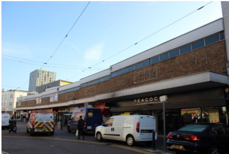
10-30 East Street is a detracting building.
